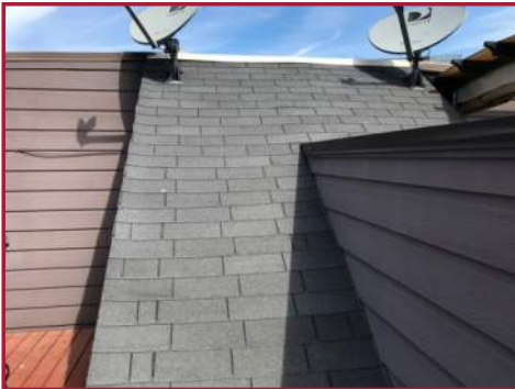
ANCILLARY ROOF #1 OVER STAIRWAY
