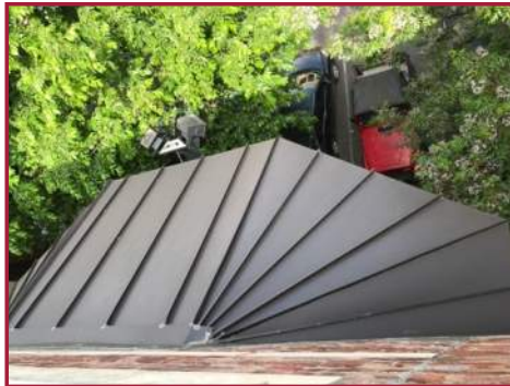
ANCILLARY ROOF #2 OVER FRONT BAY WINDOWS
