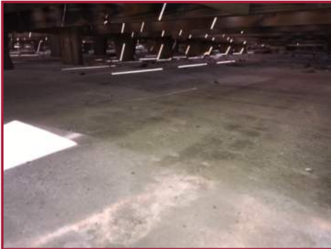
FLAT ROOF UNDER DECK
