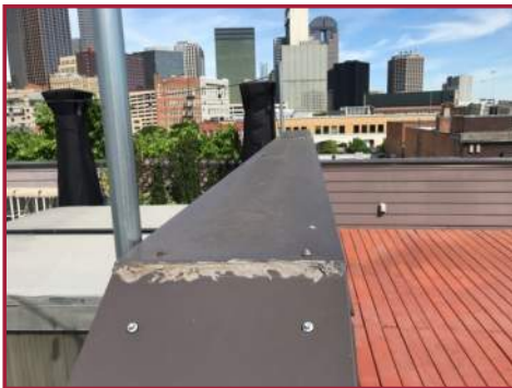
CAP FLASHING ON PARAPET WALL
