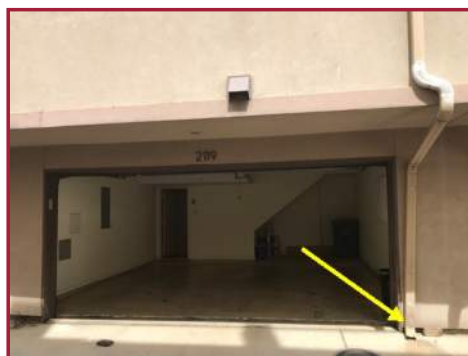
ROOF DRAIN EXIT ONTO ALLEYWAY
