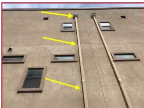
ROOF SCUPPER AND DOWNSPOUT TO ROOF DRAIN
