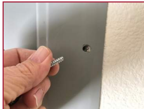
SHARP POINTED SCREWS ON PANEL COVER
