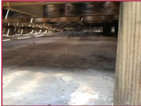
FLAT ROOF UNDER DECK
