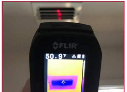
AMBIENT TEMPERATURE AT UPSTAIRS HVAC SUPPLY VENT DURING TEST
