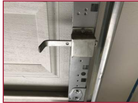
MANUAL LOCK SHOULD BE DISABLED OR REMOVED
