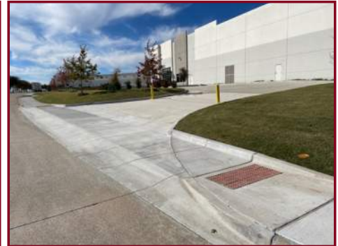
PARKING LOT EAST APPROACH
