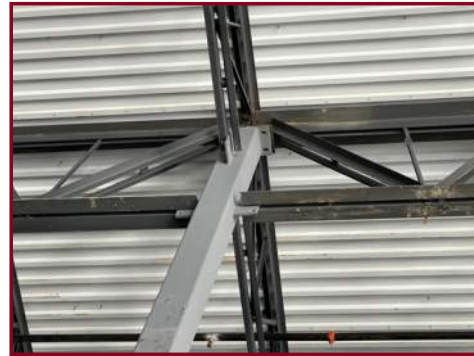
GIRDER COLUMN CONNECTIONS
