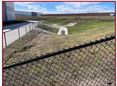
NORTH DETENTION POND
