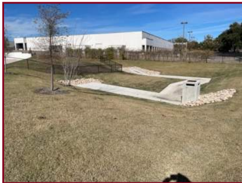
EAST DETENTION POND
