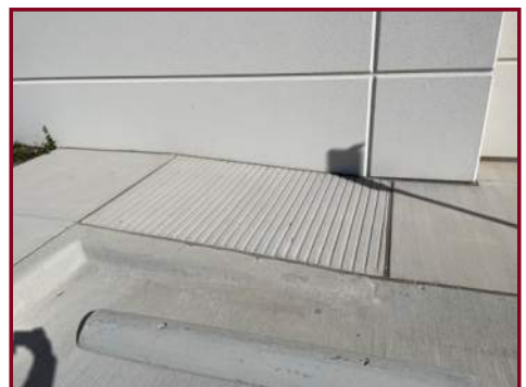
WEST DRIVE HANDICAP RAMP
