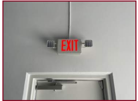
TYPICAL EXIT SIGN AND EMERGENCY LIGHTING
