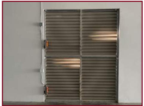
SOUTH WALL VENT
