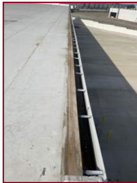
ROOF GUTTER ON EAST SIDE
