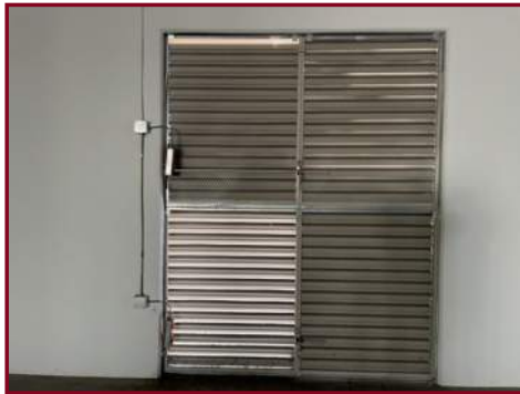
NORTH WALL VENT
