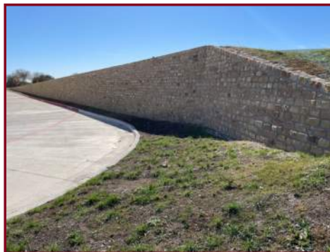
WEST RETAINING WALL
