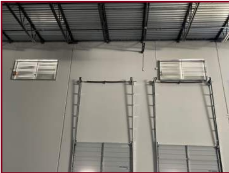
EAST WALL VENTS
