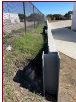
EAST RETAINING WALL
