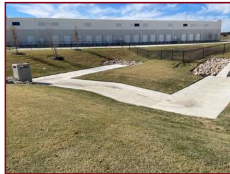
EAST DETENTION POND
