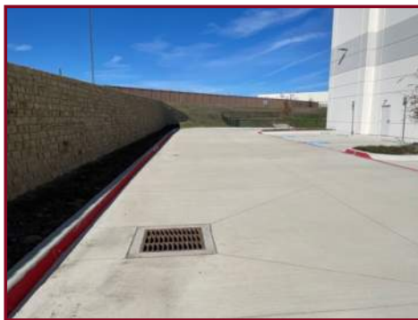
WEST DRIVE STORM DRAIN
