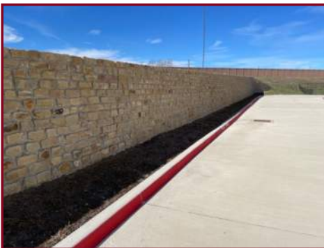
WEST RETAINING WALL
