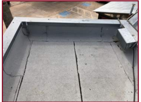
CAP FLASHING ON ROOF
