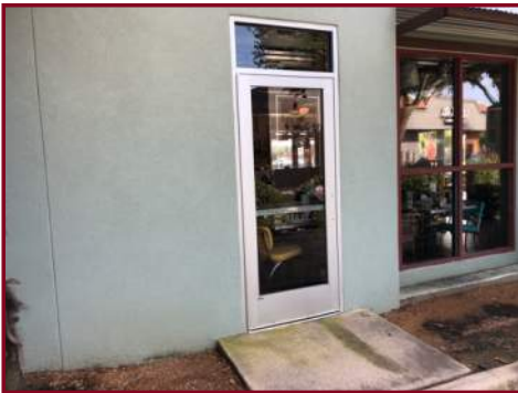
DINING AREA EMERGENCY EXIT DOOR
