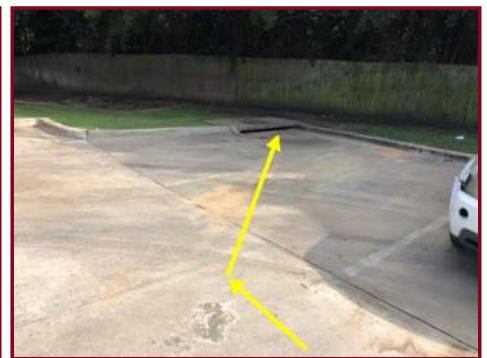
STORM DRAIN AT SOUTHEAST CORNER OF PARKING LOT
