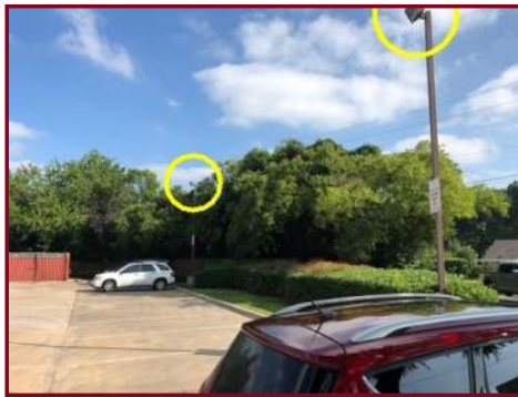
POLE MOUNTED FIXTURES
