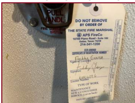
KITCHEN VENT HOOD PULL STATION INSPECTION TAG
