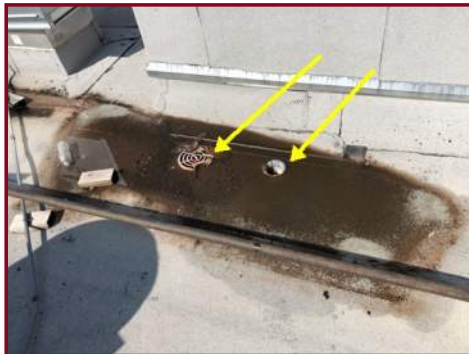
ROOF DRAIN AND OVERFLOW
