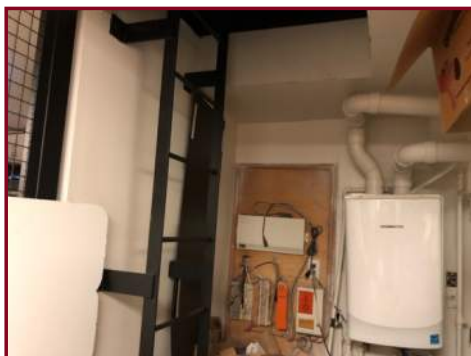
ROOF ACCESS LADDER
