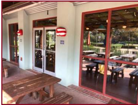
OUTDOOR DINING ENTRANCE AND GLAZING
