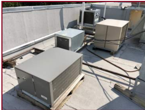
COOLER COMPRESSORS
