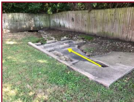
STORM WATER OUTLET AT SOUTHEAST CORNER OF PROPERTY
