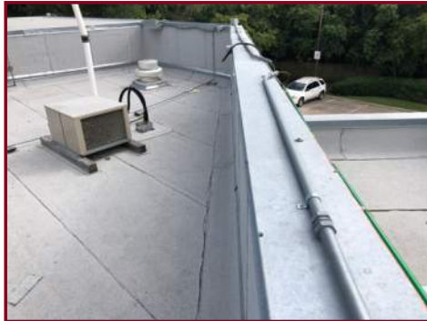
CAP FLASHING ON ROOF
