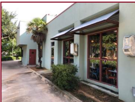
EAST ELEVATION AND GLAZING
