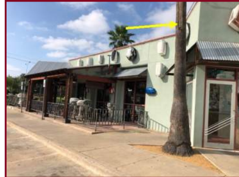
THE PALM TREE AT THE MAIN ENTRANCE APPEARS TO HAVE DIED
