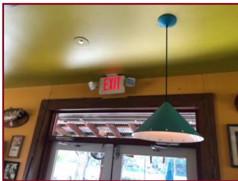
TYPICAL EXIT SIGN AND EMERGENCY LIGHTING
