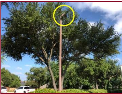
POLE MOUNTED FIXTURES
