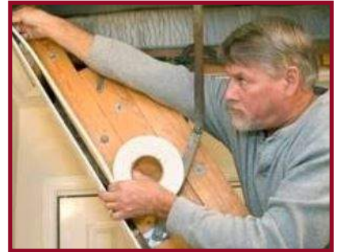
ATTIC LADDER WEATHERSTRIPPING ILLUSTRATION
