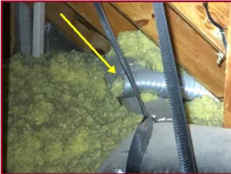
MECHANICAL EXHAUST VENTS EXIT INTO ATTIC
