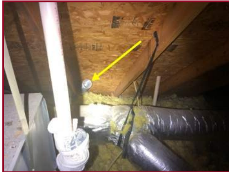
MECHANICAL EXHAUST VENTS EXIT INTO ATTIC
