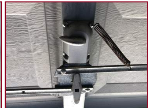
MANUAL LOCK SHOULD BE DISABLED OR REMOVED
