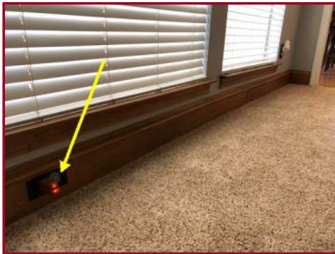
REVERSE POLARITY IN RECEPTACLE ON WEST WALL OF LIVING ROOM
