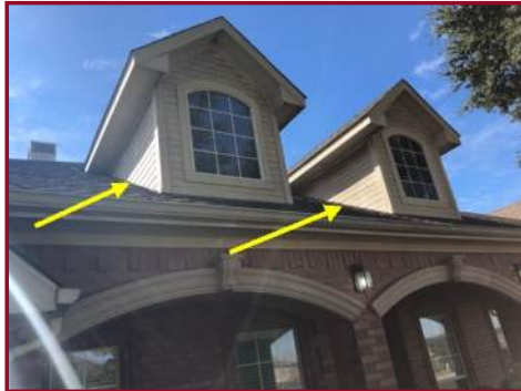
SIDEWALL VENEER IN CONTACT WITH ROOF
