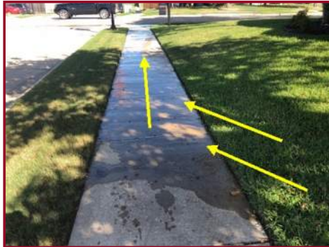
WATER LEAKING FROM SEWER DOWN SIDEWALK
