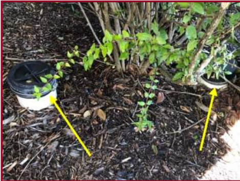
SEWER CLEANOUTS IN EAST FLOWERBED
