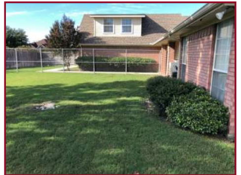
MARGINAL DRAINAGE ON WEST SIDE OF HOUSE
