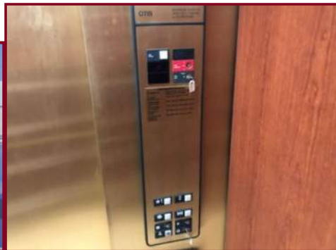
ELEVATOR CONTROLS
