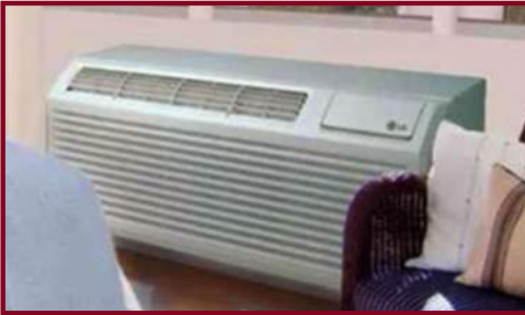
TYPICAL PACKAGED ROOM HVAC UNIT
