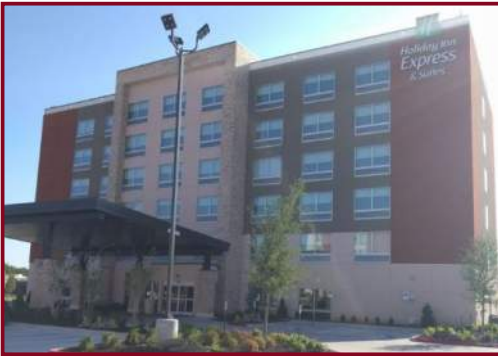
POLE MOUNTED FIXTURES
